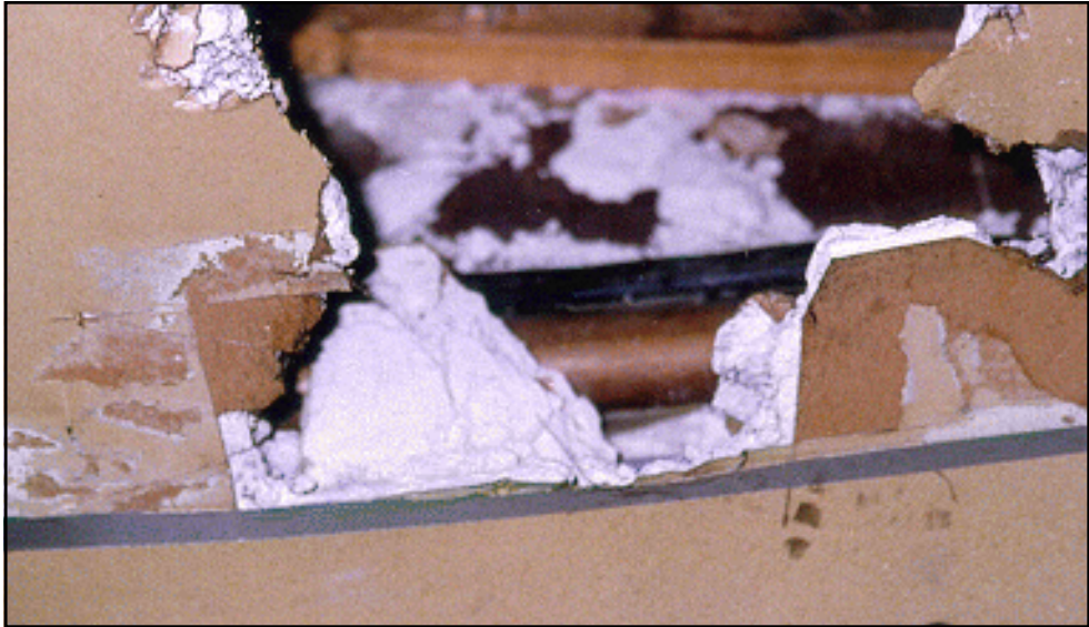
FIGURE 4-2 Subfloor Penetration
